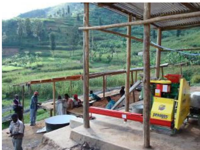
Coffee Pulping Unit installed in Rwanda. (Courtesy of J. Schluter)
